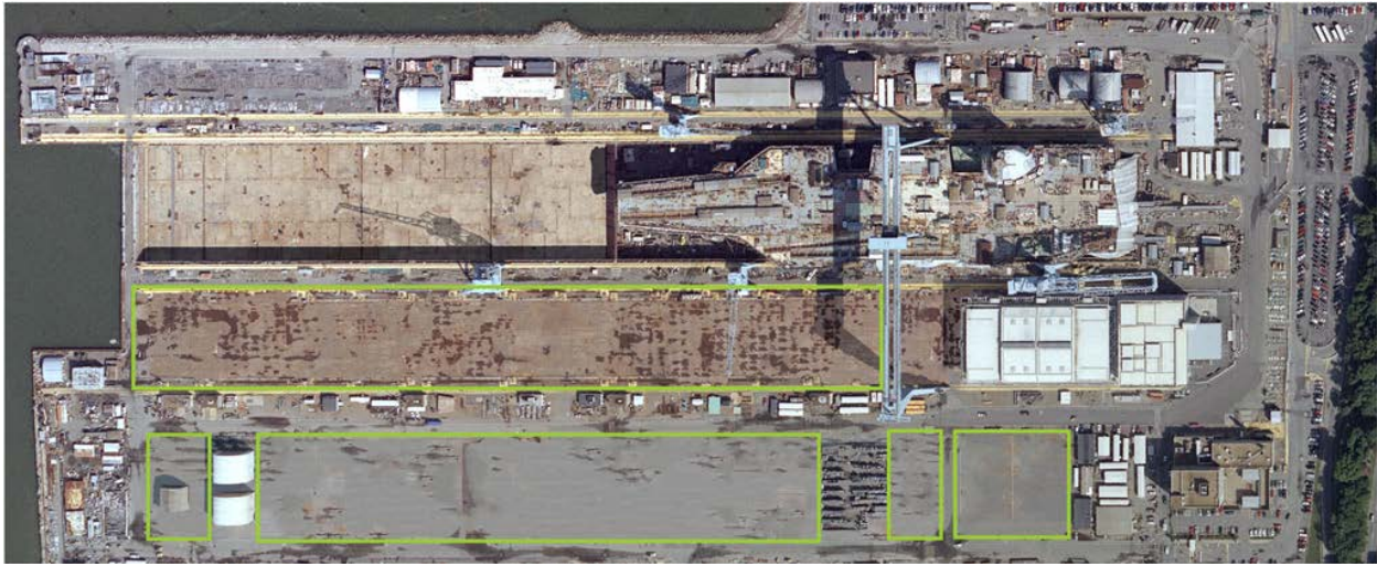
Figure 3: Lay-Down Area Cleared of Material/Units
